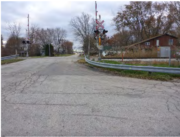
Photo 1: View of study area illustrating Rourke Line Road, facing south
