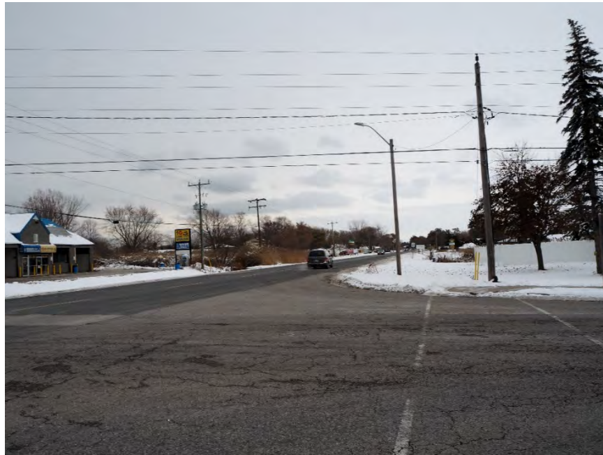
Plate 9: County Road 22 looking east from Rourke Line Road
