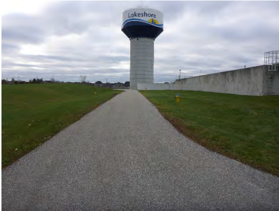
Photo 25: View of existing WPCP illustrating extensive terraforming, facing south
