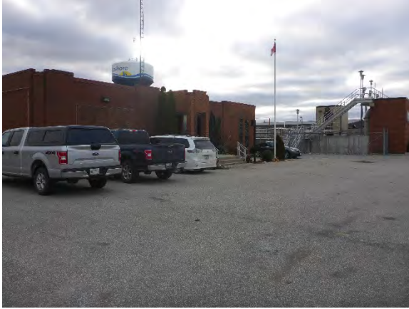
Photo 21: View of existing WPCP, facing southeast
