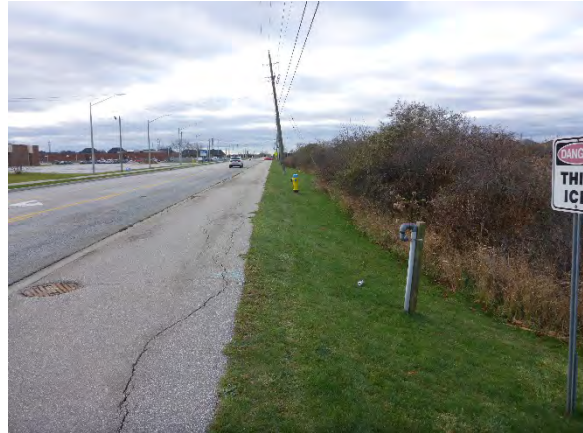
Photo 10: View of study area illustrating road ROW and buried infrastructure, facing south
