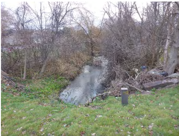
Photo 19: View of constructed ditch alongside rail line, facing east
