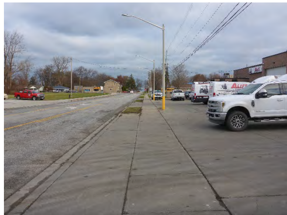
Photo 16: View of study area illustrating road ROW, facing north
