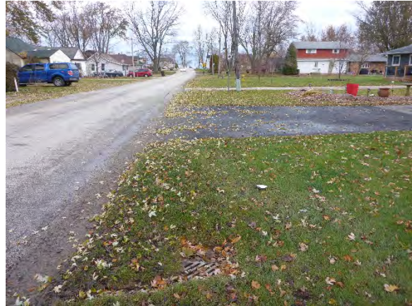
Photo 18: View of study area illustrating road ROW and buried infrastructure, facing north
