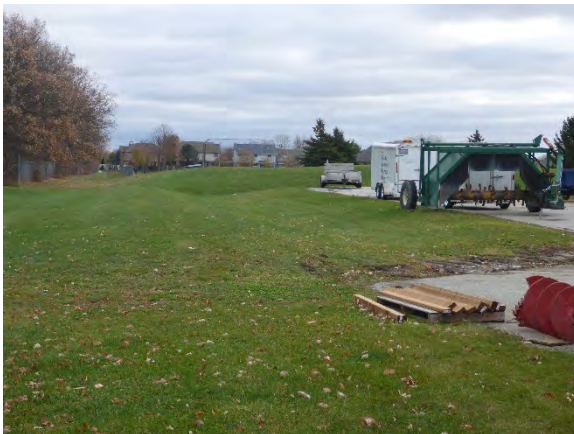
Photo 23: View of existing WPCP illustrating extensive terraforming, facing east
