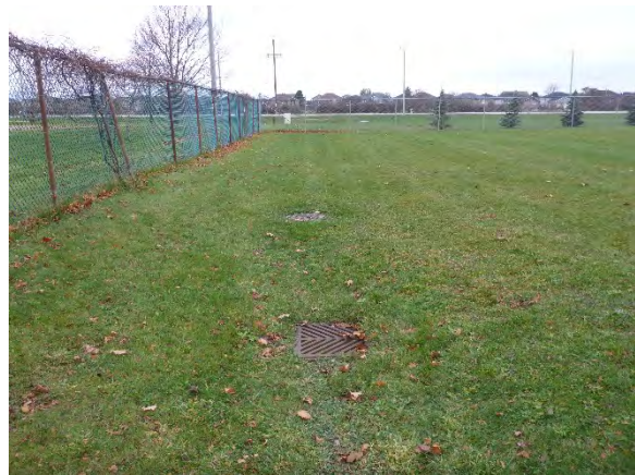
Photo 28: View of buried infrastructure within the existing WPCP, facing west
