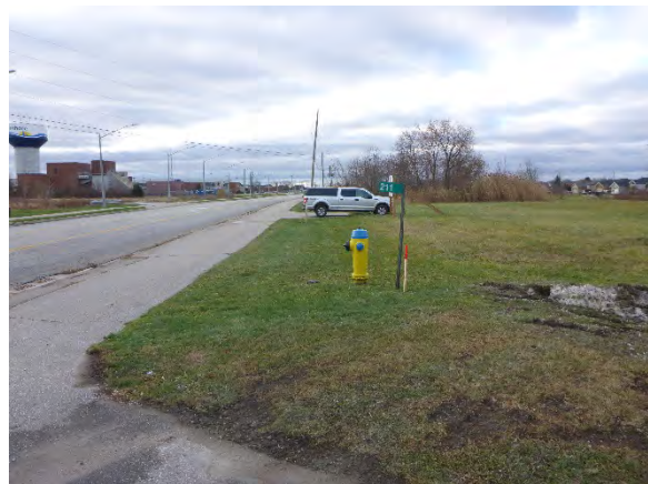
Photo 8: View of study area illustrating road ROW and buried infrastructure, facing south
