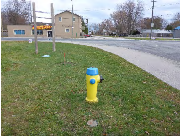
Photo 5: View of study area illustrating road ROW and buried infrastructure, facing north
