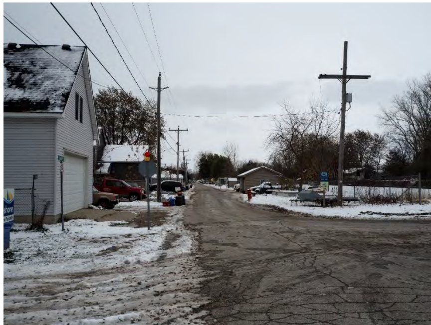
Plate 12: Caille Avenue looking east from Rourke Line Road
