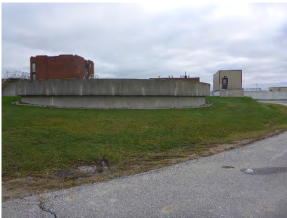
Photo 27: View of existing WPCP, facing east
