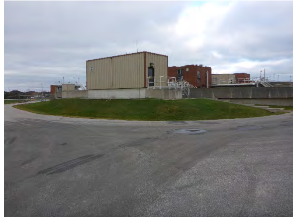
Photo 26: View of existing WPCP, facing northwest
