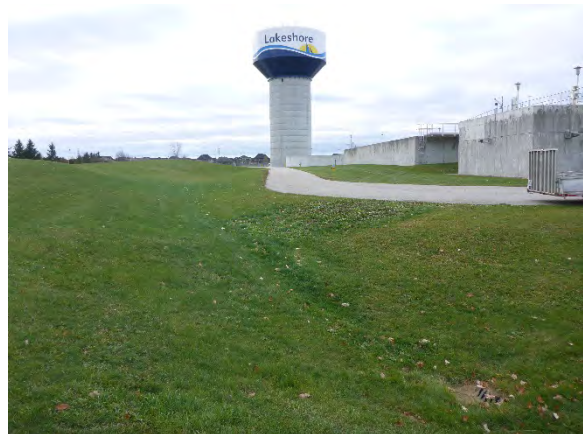
Photo 24: View of existing WPCP illustrating extensive terraforming, facing south
