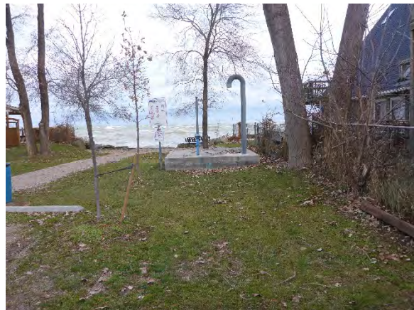
Photo 20: View of study area illustrating buried infrastructure, facing north
