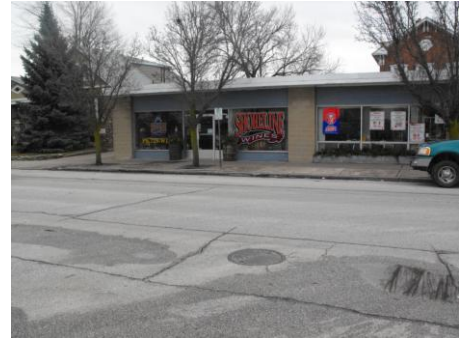
Existing Building Façade
