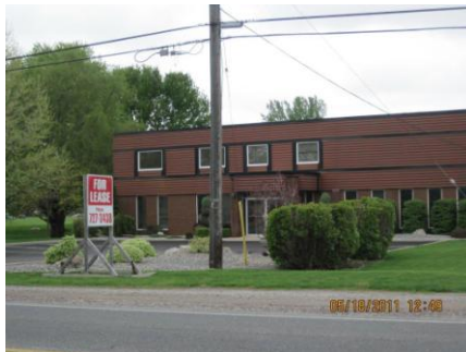
Vacant Commercial Building
