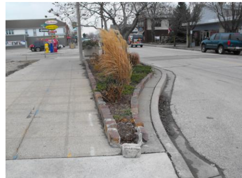
Existing Brick Planter
