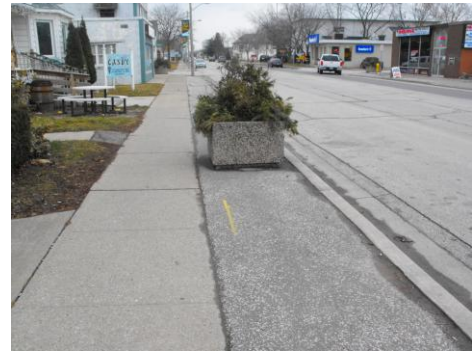
Existing Boulevard Treatment
