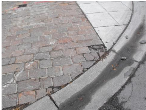
Existing Brick Pavers
