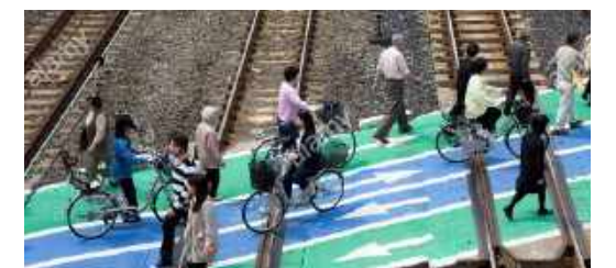
Example of Improved Railway Crossing
