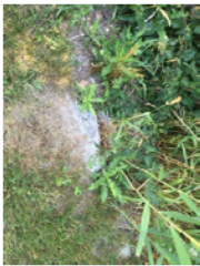
6) CONCRETE IN GRASS
