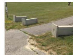
6) BOLLARDS AT WEST PARKING LOT
