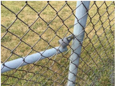
10) PARKING LOT FENCE REPAIRS
