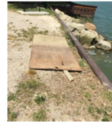
7) PATH AT BREAKWALL
