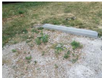
3) GRAVEL PARKING AREA
