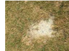
6) CONCRETE IN TURF
