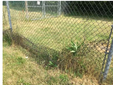
11) PARK FENCE REPAIRS
