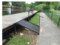
9) RAMP TO DOCK
