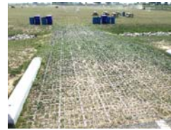
4) REINFORCED TURF ACCESS ROAD
