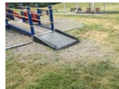
7) RAMP TO PLAY STRUCTURE
