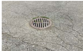
2) PARKING LOT CATCH BASIN
