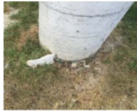
1) PARKING LOT LIGHTING
