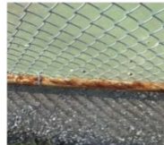
11) TENNIS COURT FENCING
